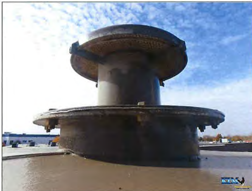
Photo No. 20 Vent/finial
