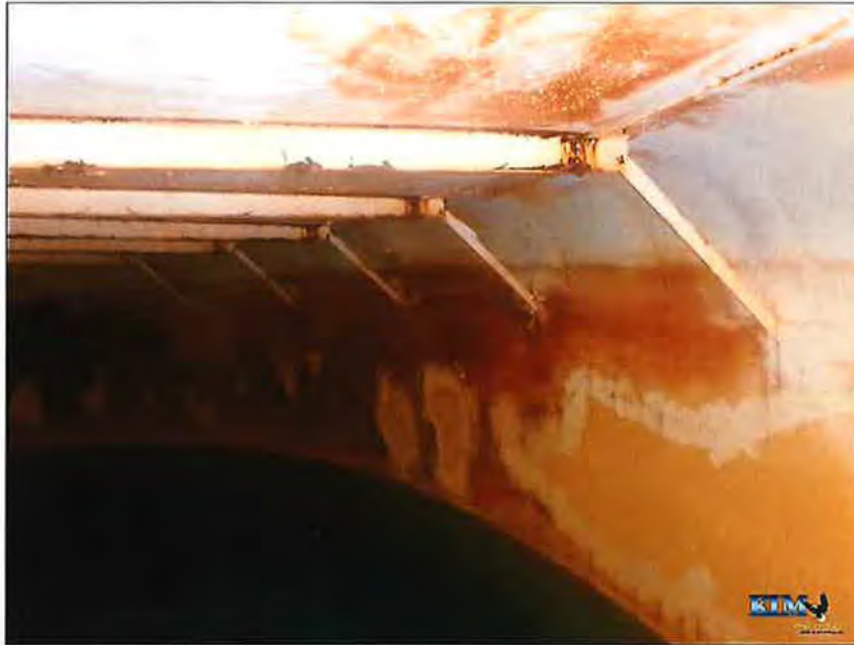
Photo No. 7 Roof and upper shell
