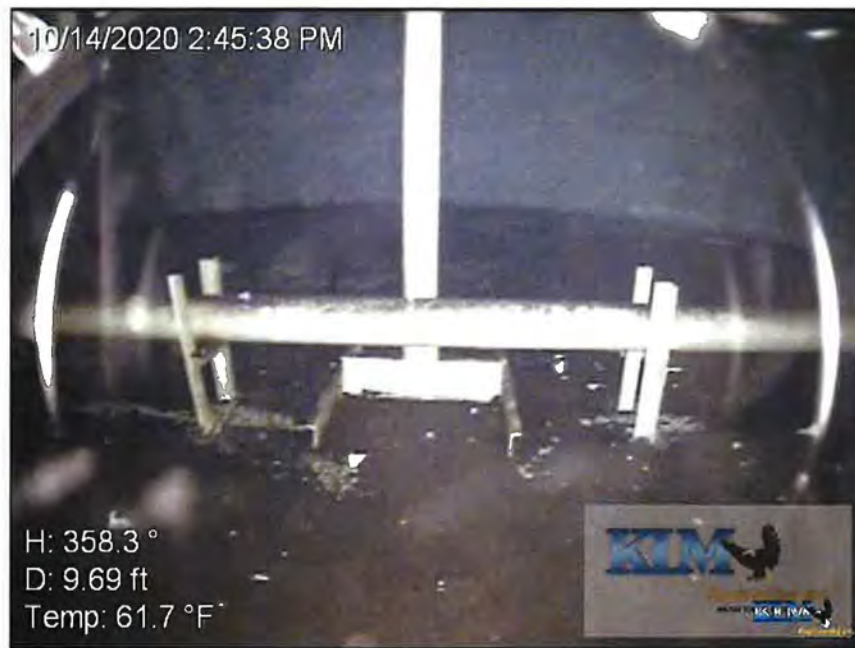
Photo No. 17 Condition of floor, center column and fill pipe with bracing
