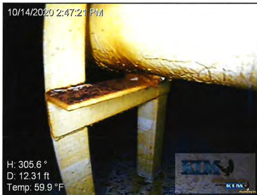
Photo No. 18 Fill pipe straddled in bracing
