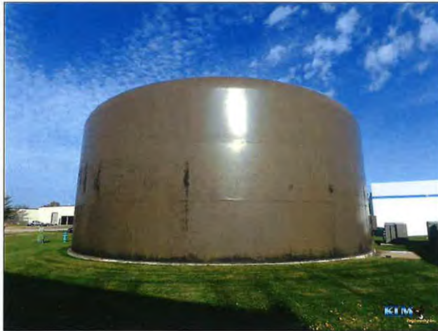
Photo No. 1 Overall view of the reservoir
