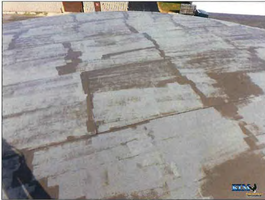
Photo No. 21 Roof coating condition
