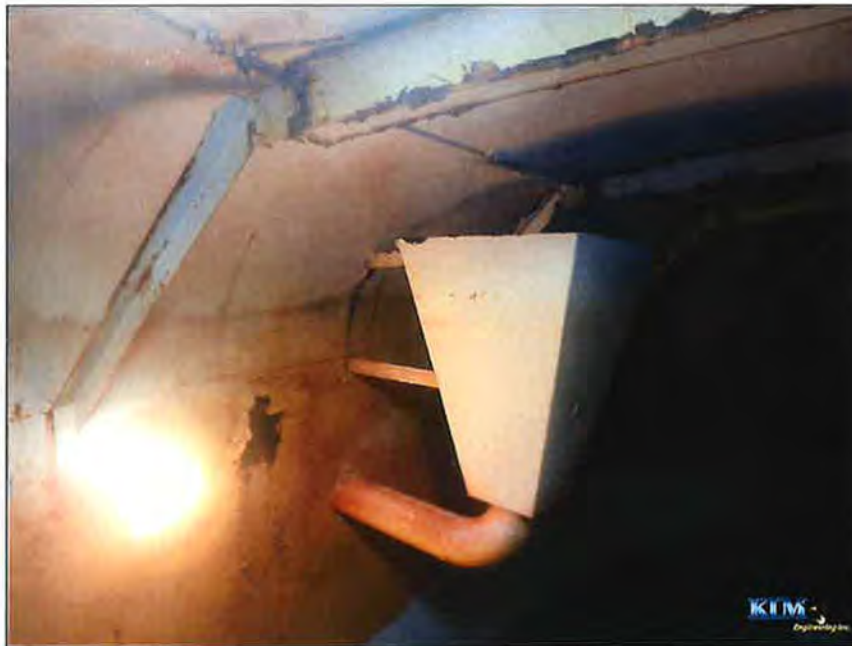
Photo No. 5 Overflow weir and conditions
