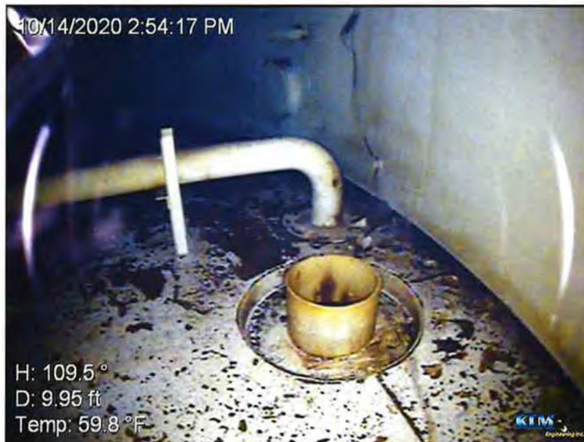
Photo No. 16 Discharge and conditions
