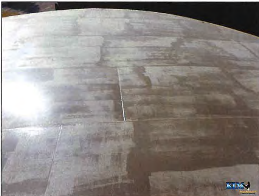
Photo No. 22 Roof coating condition
