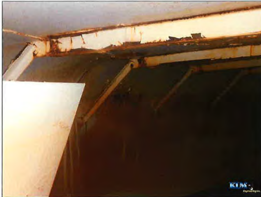
Photo No. 3 Condition of roof structure
