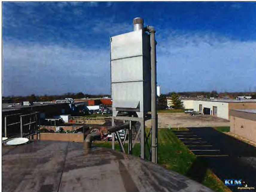
Photo No. 24 Abandoned aerator
