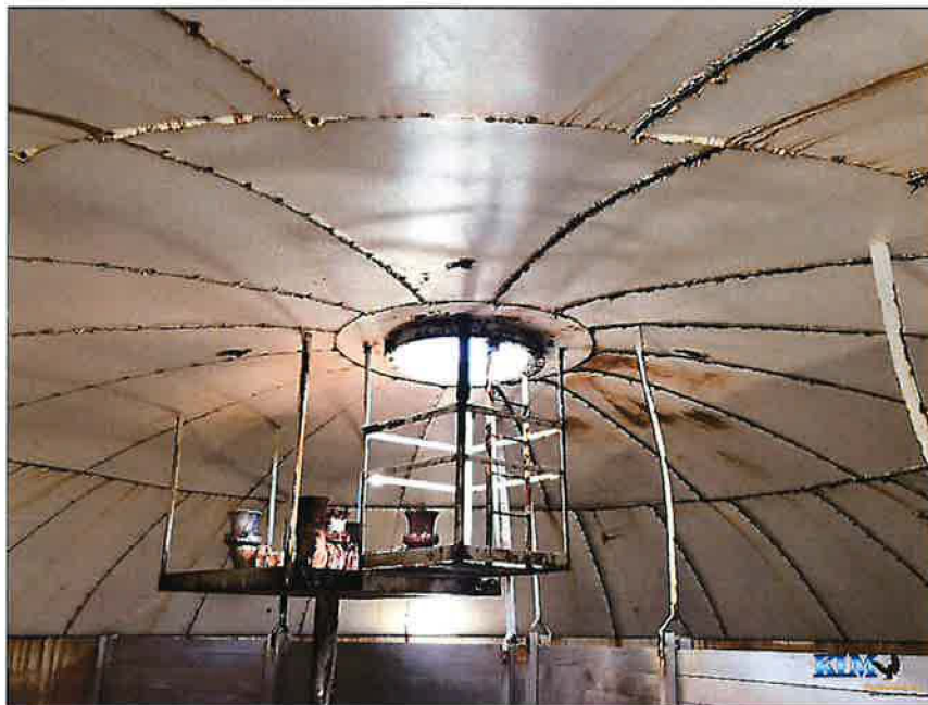
Photo No. 2 Overall roof condition, note center fill de-fuser and inspection platform
