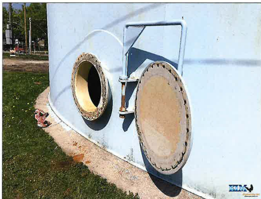
Photo No. 36 Shell manway and foundation conditions
