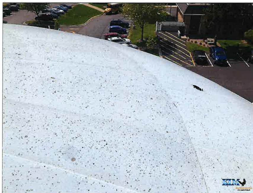
Photo No. 28 Overall roof conditions
