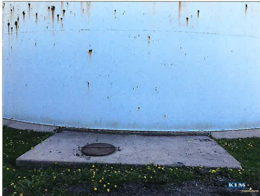
Photo No. 41 Valve pit roof and access manway
