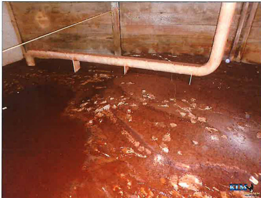
Photo No. 24 Floor conditions and inlet pipe
