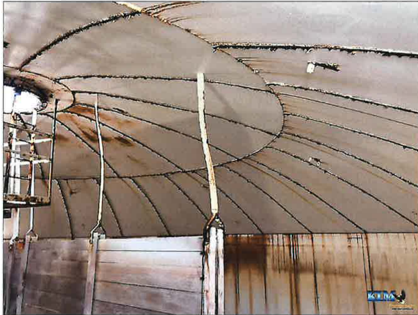
Photo No. 15 Baffle wall connection to roof
