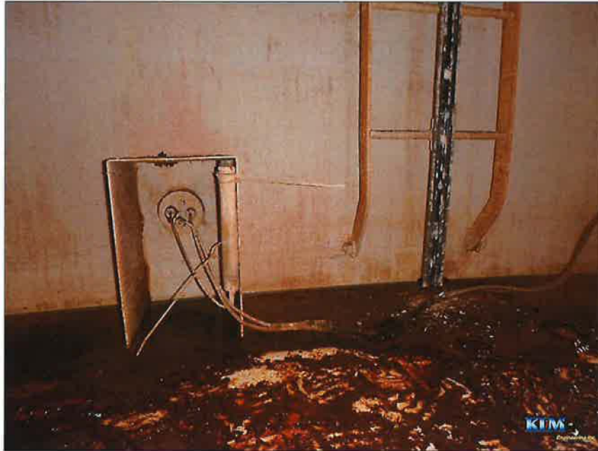
Photo No. 23 C.P. penetration on shell and floor conditions
