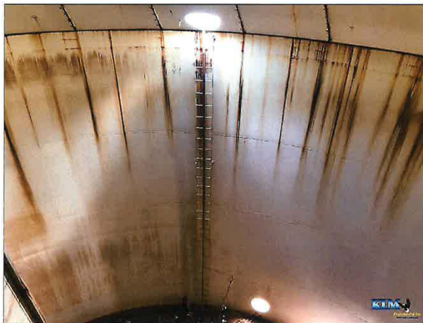
Photo No. 18 Overall condition of shell
