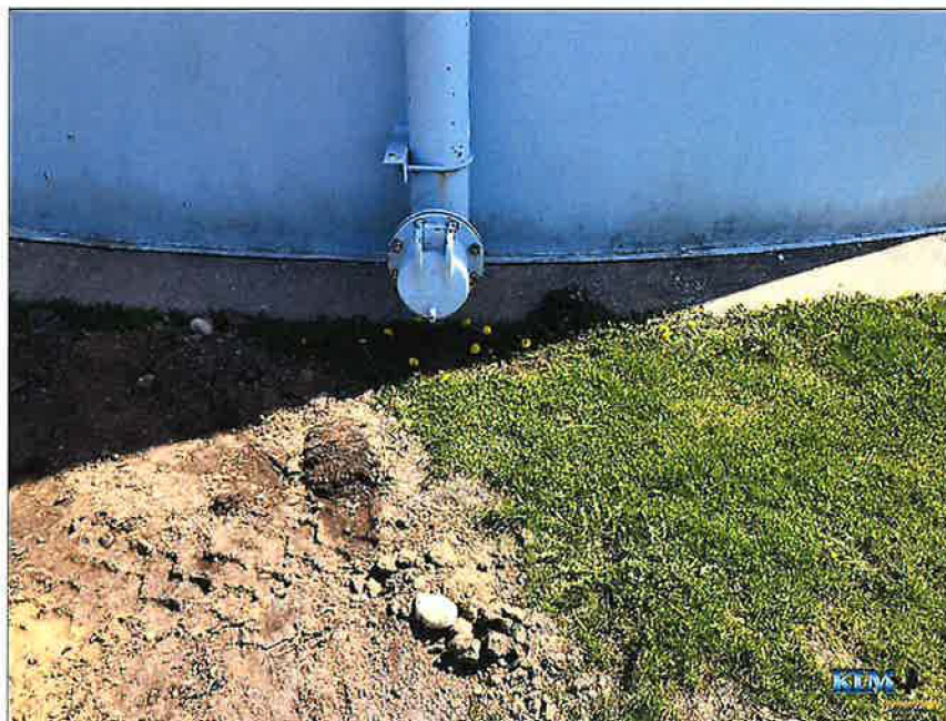
Photo No. 38 Overflow discharge
