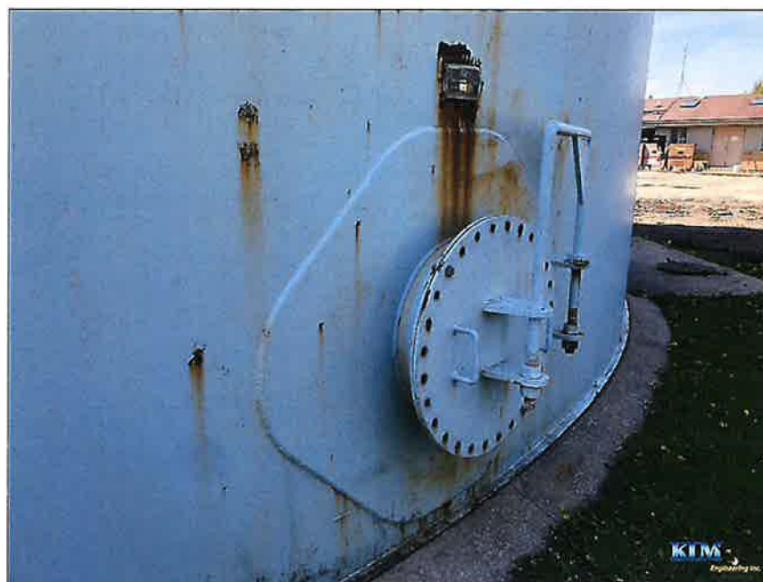
Photo No. 34 Shell manway
