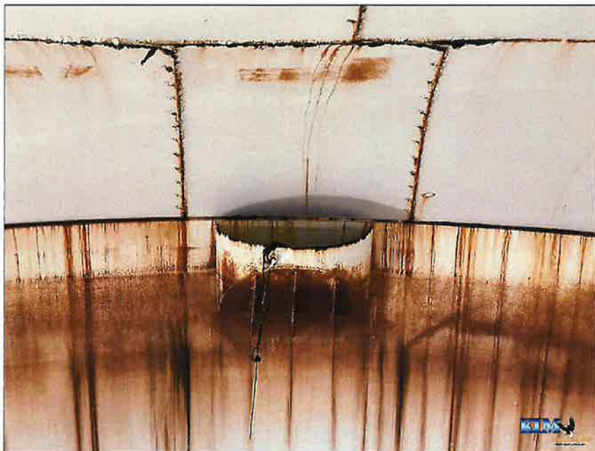
Photo No. 8 Overflow weir box and roof/shell condition
