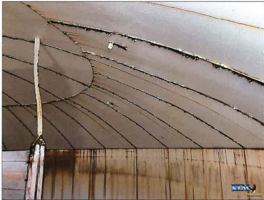
Photo No. 3 Roof condition
