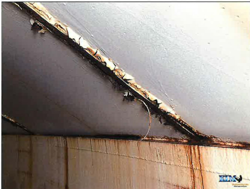
Photo No. 16 Roof to shell connection and conditions
