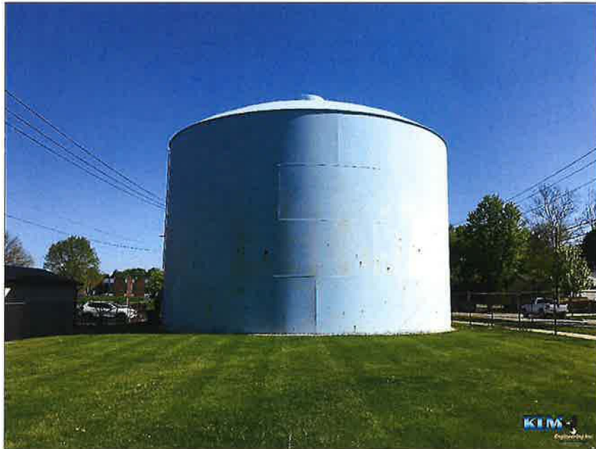
Photo No. 1 Overall view of reservoir
