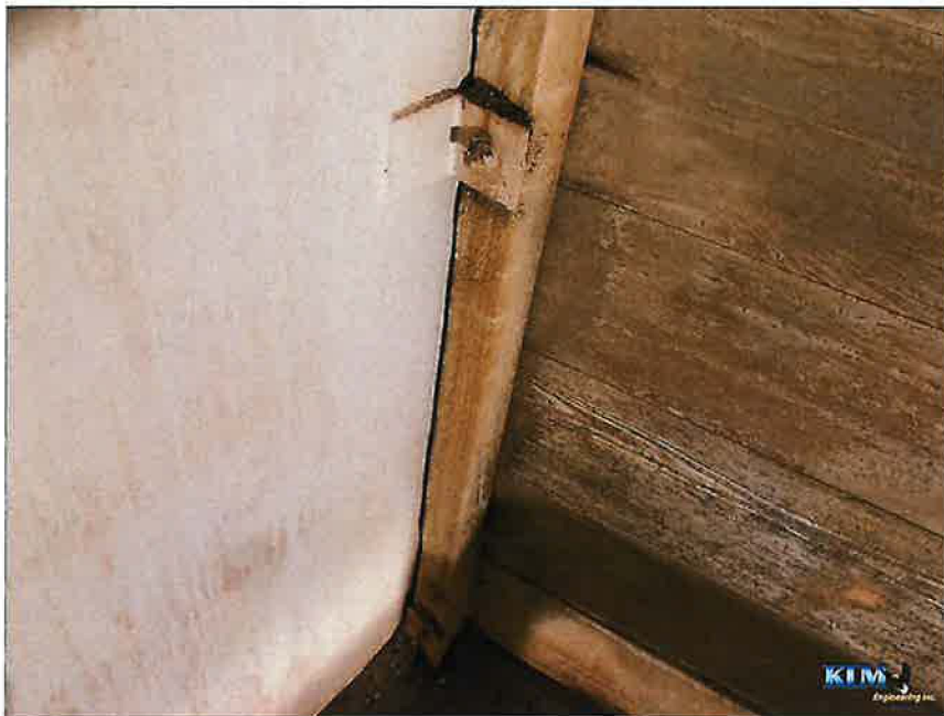
Photo No. 14 Baffle wall connection to reservoir shell
