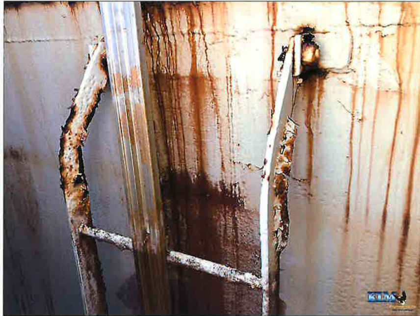
Photo No. 17 Ladder condition at top of shell
