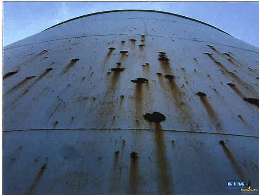
Photo No. 33 Shell coating condition
