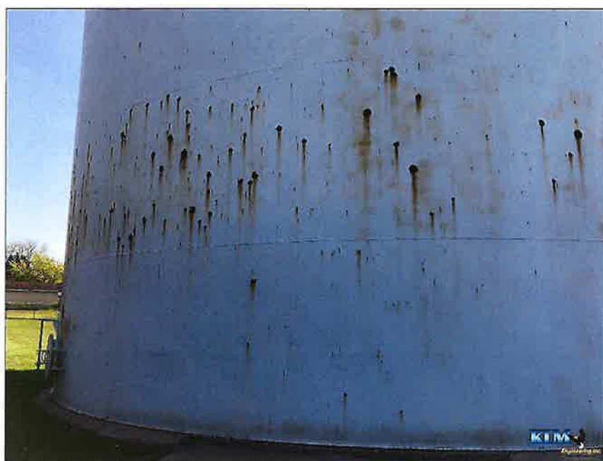
Photo No. 40 Shell coating condition
