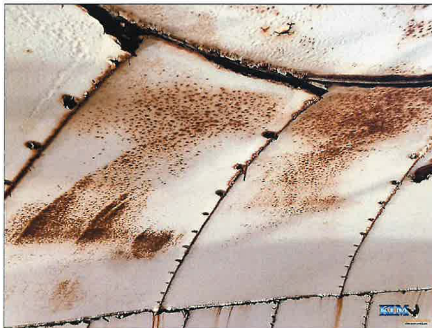
Photo No. 4 Roof condition
