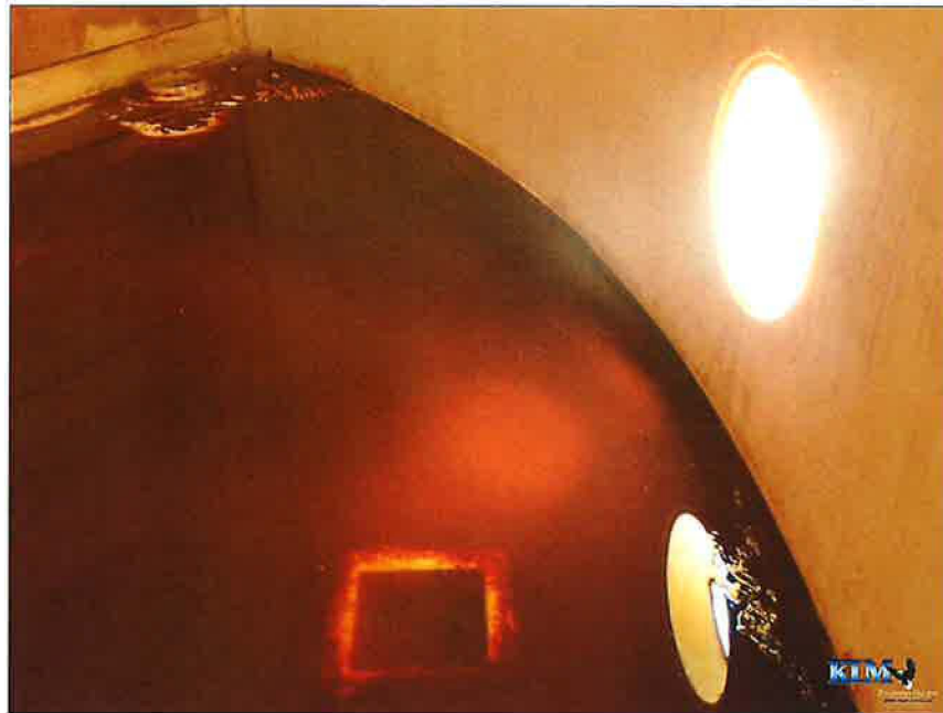
Photo No. 25 Floor conditions, note sump pit and shell manway
