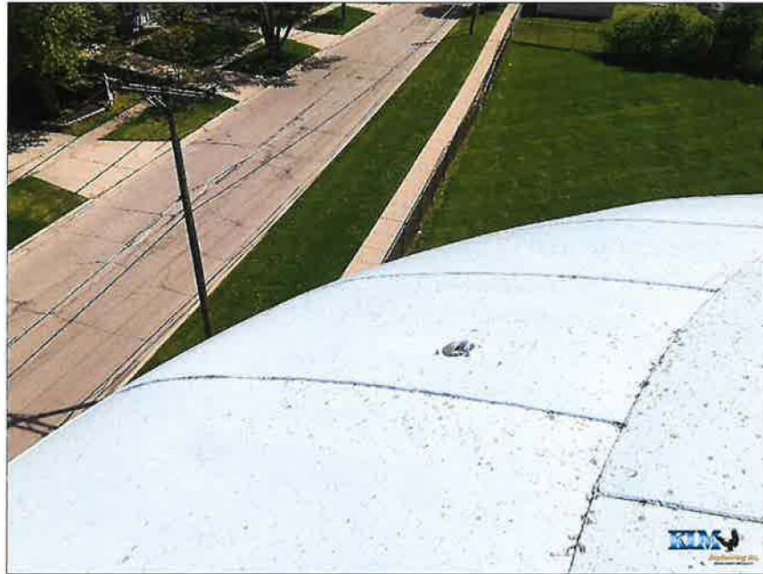
Photo No. 29 Roof conditions
