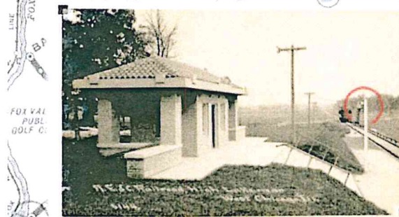
The High Lake stop was a flag station stop, meaning the conductor would stop to board passengers if a flag, or semaphore, was raised. The semaphore pole can be seen on the right side of the picture above. Passengers would pull a chain to lift the semaphore, then pull the chain again to drop the semaphore before boarding the train.
