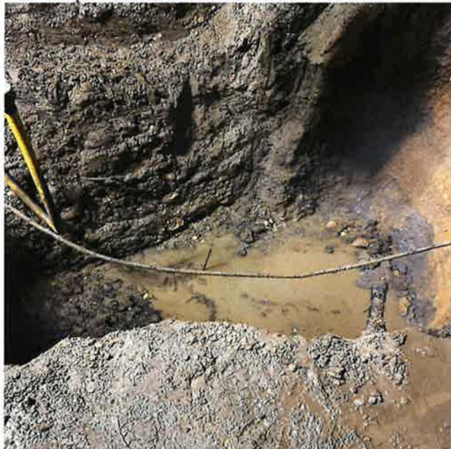
Excavation site 11/22/19 at 9:00 p.m. The depth is 18'
