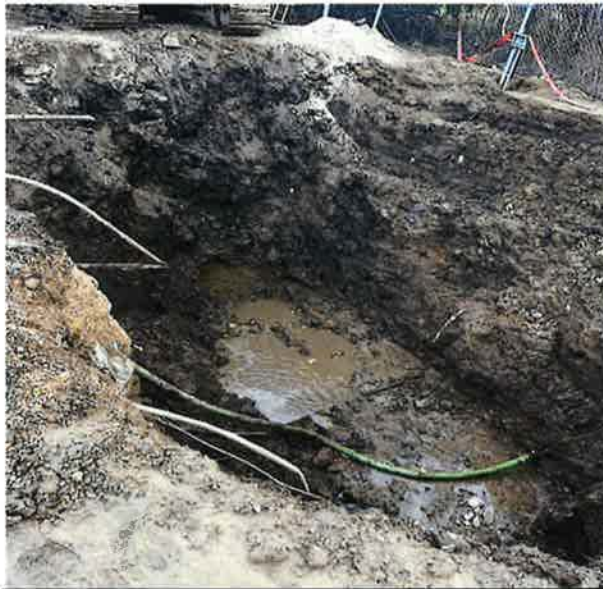
11/23/19 at 2:20p.m. The excavation is 40' x30' wide and 18' deep at this point.
