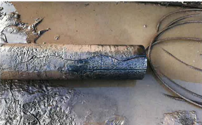
Section of watermain removed 11/25/19
